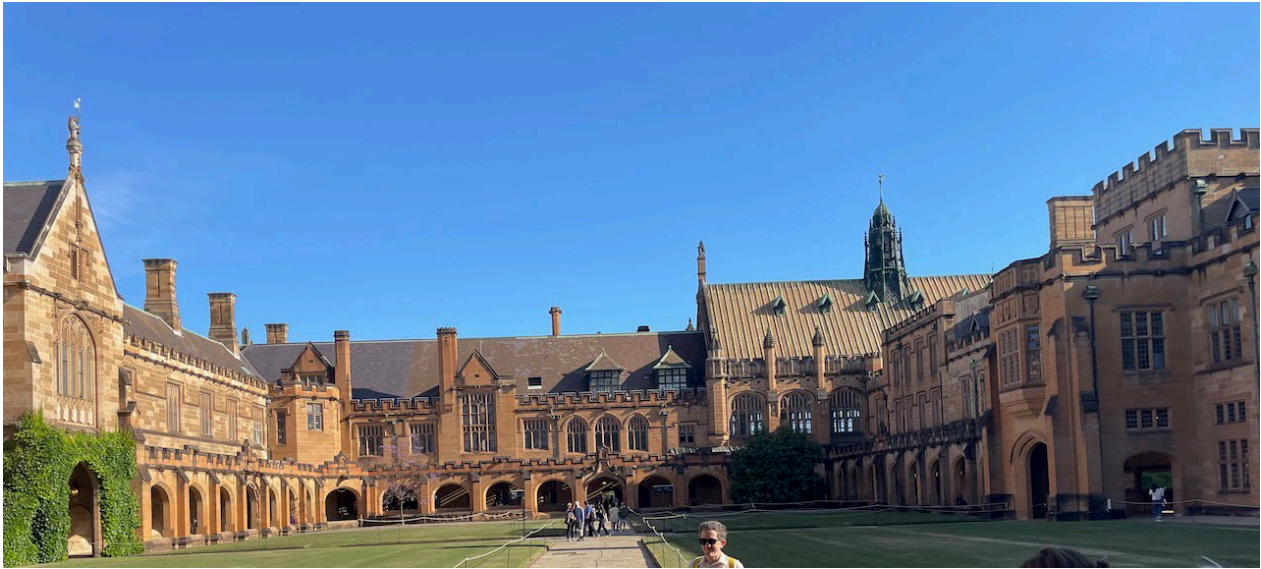
Figure 6: 2023 photograph of the Edmund Blackett 1850's designed quadrangle, completed in the 1920s Masterplan for University of Sydney by Professor Wilkinson.
